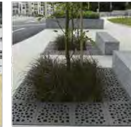
Tree grates: Powdercoated steel with patterned perforations
