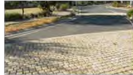
Shared zone pavement texture: sand coloured set pavers to indicate pedestrian crossing
