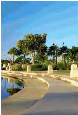
Waters edge: concrete revetment walls with some terracing to allow access to waters edge
