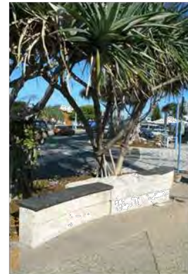
Arrival node: exposed aggregate plaza with contrasting concrete and timber shaded seating
