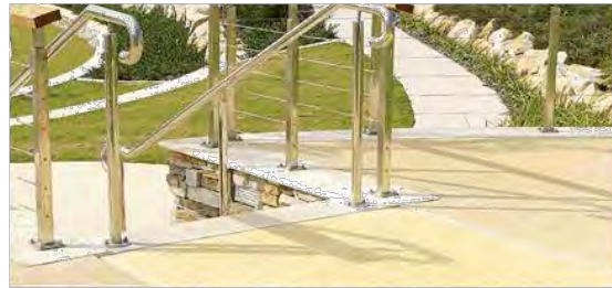
Landings and entries: grey and coloured concrete. Fittings: stainless steel railings and handrails.
