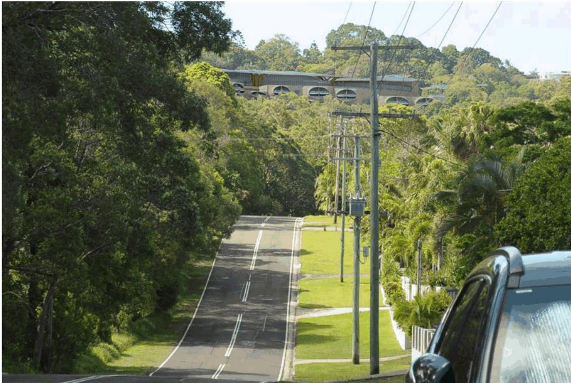
View from Cogill Rd
