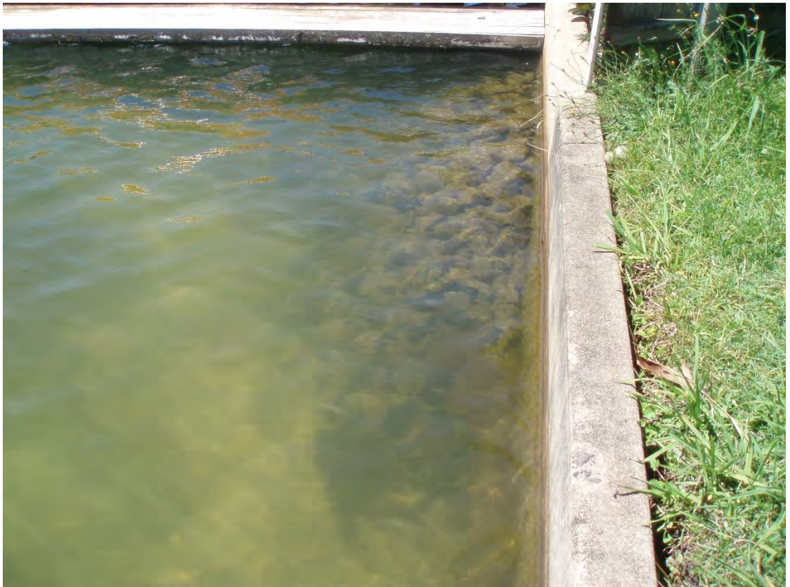
Figure 2-6 Additional Rock Scour Protection 36 Saltwater Av.
