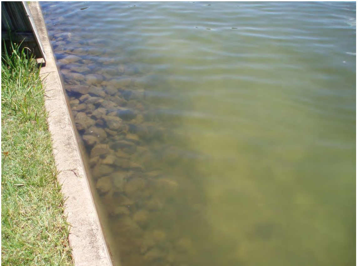
Figure 2-5 Additional Rock Scour Protection 40 Saltwater Av.
