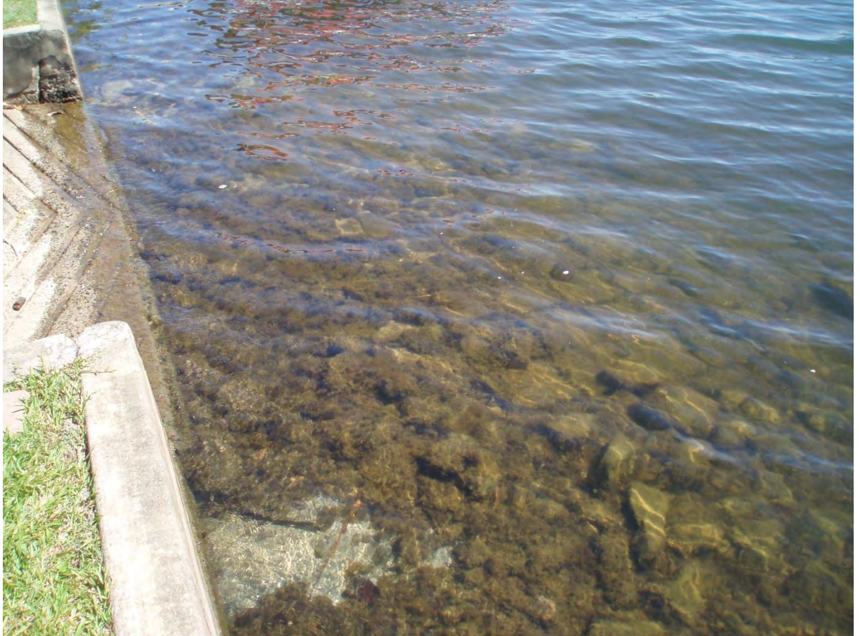
Figure 2-14 Waterside Court flexible concrete mat boat ramp
