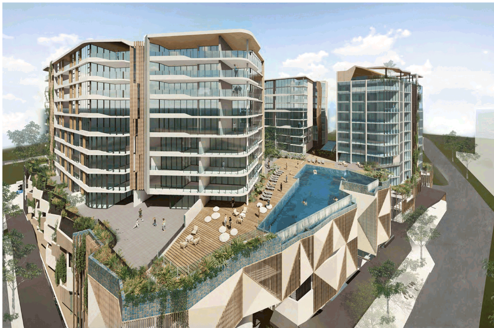
Pool and Landscaped Recreation Podium
