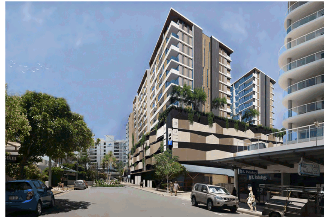
View from South-West along Smith Street
