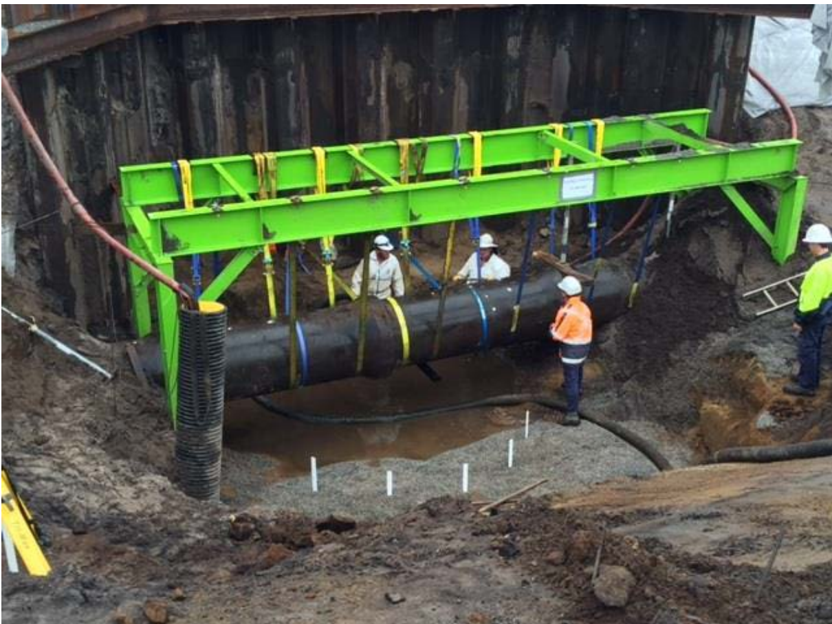
Image 2. Live sewer connection/interface works
