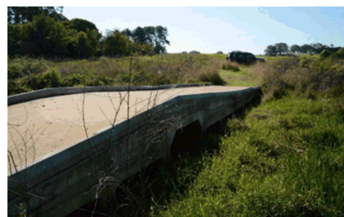
Wetland Outlet Structure
