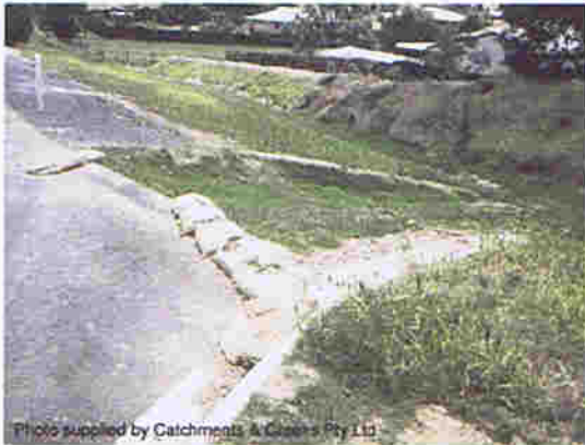
Photo 3 – Sandbags (temporary) used to control flow entry into grass chute
