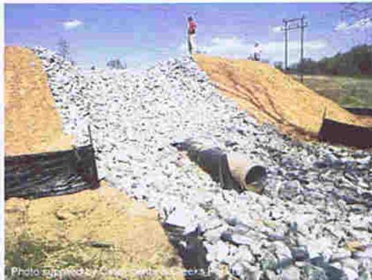
Photo 19 – Rock-lined spillway with well-defined crest profile
