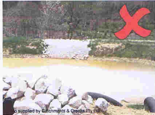
Photo 20 – Rock-lined spillway with poorly defined crest profile
