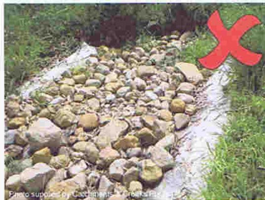
Photo 23 – Rounded rock can be significantly less stable than angular, fractured rock, especially when placed on steep slopes
