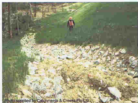
Photo 17 – Permanent, rock-lined batter chute
