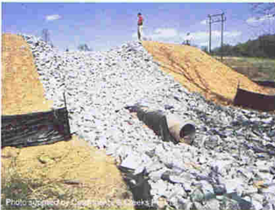
Photo 5 – Spillway chute with well-defined inlet profile
