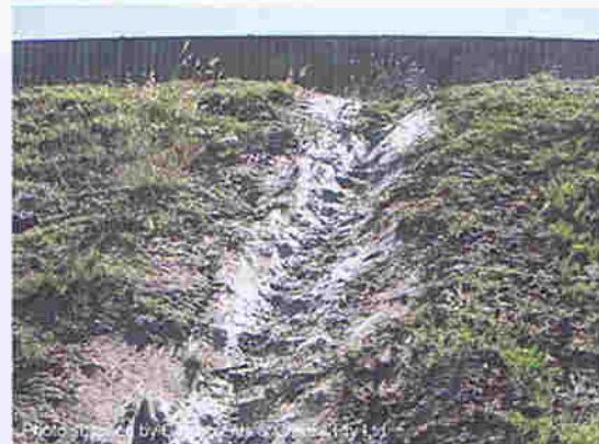
Photo 2 – Temporary batter chute lined with filter cloth
