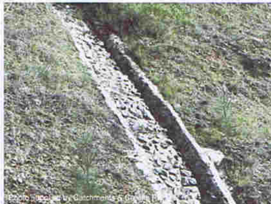
Photo 1 – Permanent, grouted-stone batter chute
