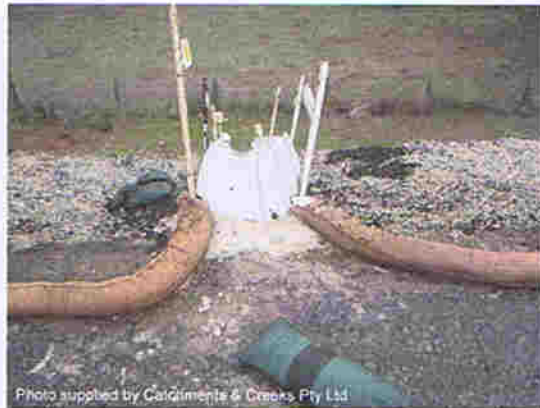
Photo 4 – Geotextile socks used to control flow entry into temporary batter chute
