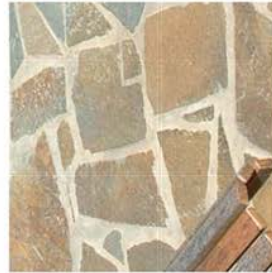
Random Porphyry stone paving
