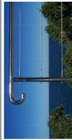
Marine grade stainless steel handrail and wire balustrading. Wickham Point, Caloundra
