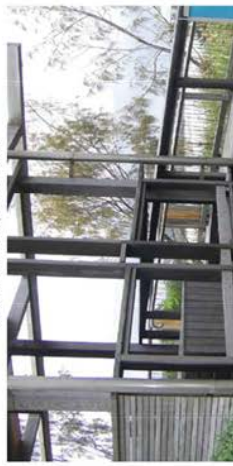
Marine grade stainless steel handrail and wire balustrading. Wickham Point, Caloundra
