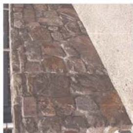
Mixed stone retaining wall, Bulcock Beach, Caloundra
