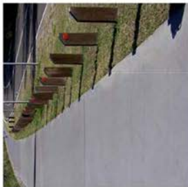
200 x 75 x 85 hardwood timber bollard
