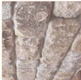
Sandstone retaining wall
