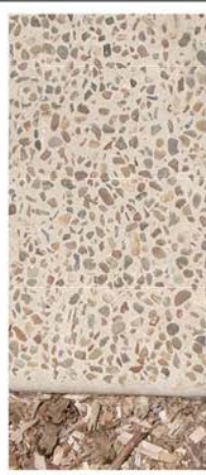
Light-exposed coloured concrete with Mary River aggregate. Leach Park, Golden Beach
