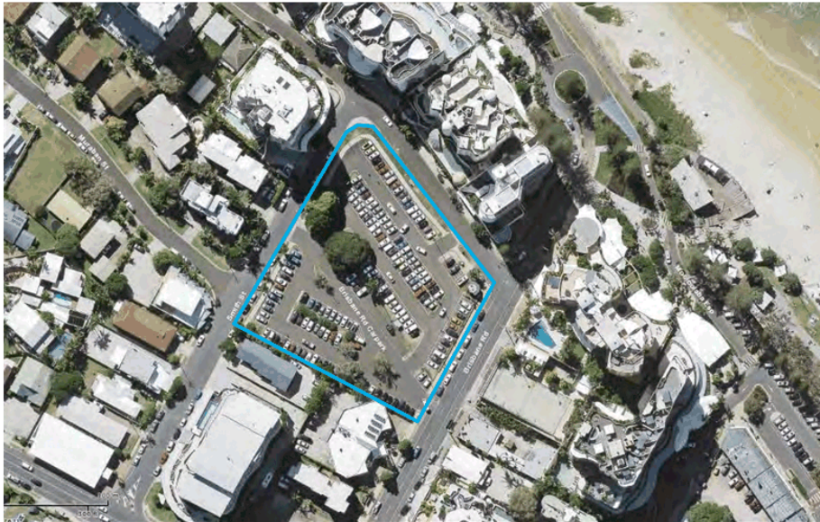
Figure 2: site aerial view
