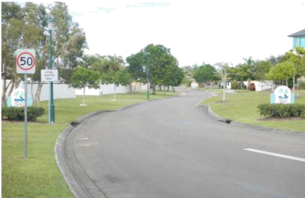
Photograph 3: View south along Sir Joseph Banks Drive approximately 50m south of Nelson Street. Kerb extensions can be seen beyond the 'Local Traffic Only' sign.
