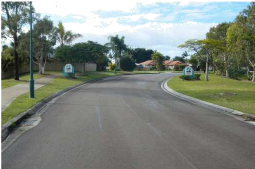
Photograph 8: View looking east along Sir Joseph Banks approaching the intersection with Lamerough Parade.
