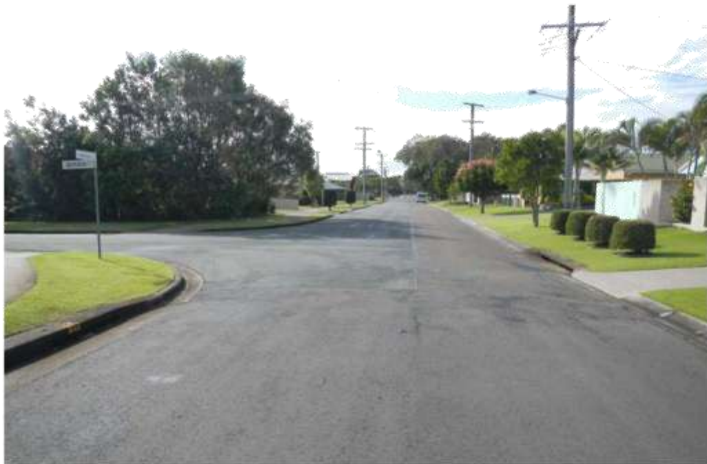
Photograph 12: View looking east along Lamerough Parade approaching the intersection with Moorshead Avenue.
