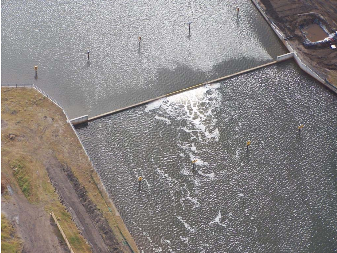
Figure 6: Lake kawana Weir 2007
