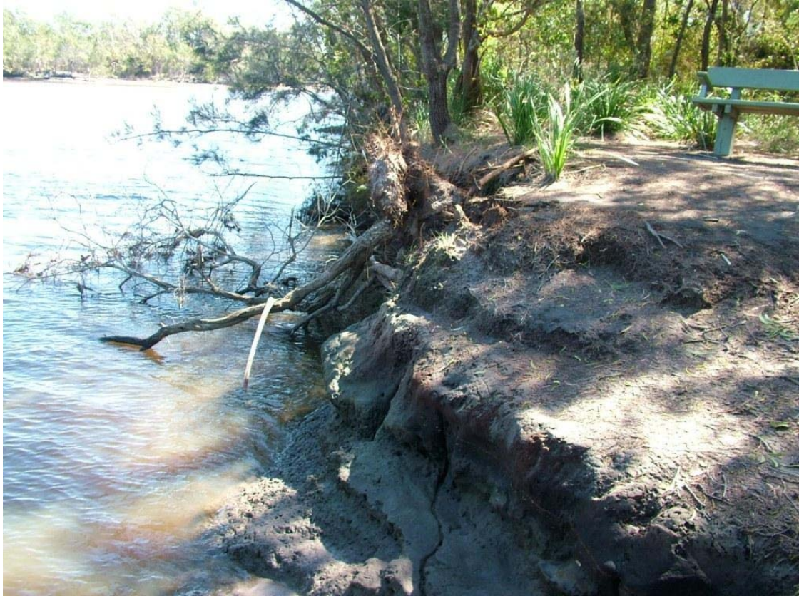
Figure 5: Typical bank erosion
