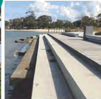
Hard terraced edge hard terracing for erosion control, spectator seating and easy access to waters edge
