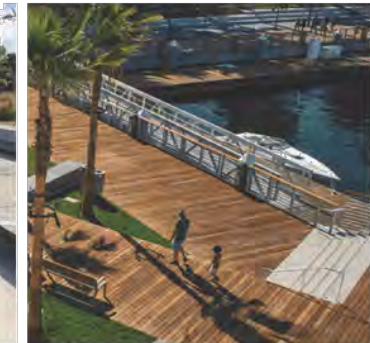
Wharf boardwalk edge over-water boardwalk with active frontage and access to marina pontoons
