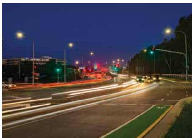
Evans St Upgrade Maroochydore, increased road safety and improved traffic flow
