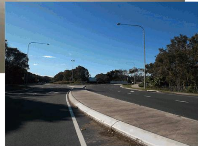
VP08b - David Low Way, existing roundabout
