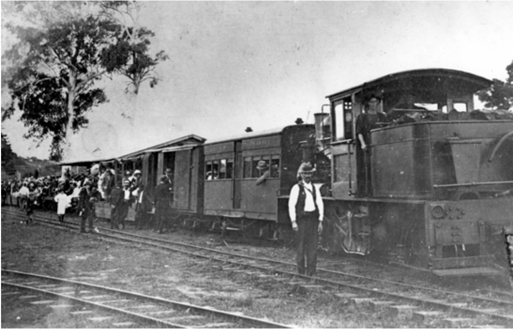
Figure 28: Buderim tram terminus showing Brisbane day trippers c1920 (Sunshine Coast Library).
