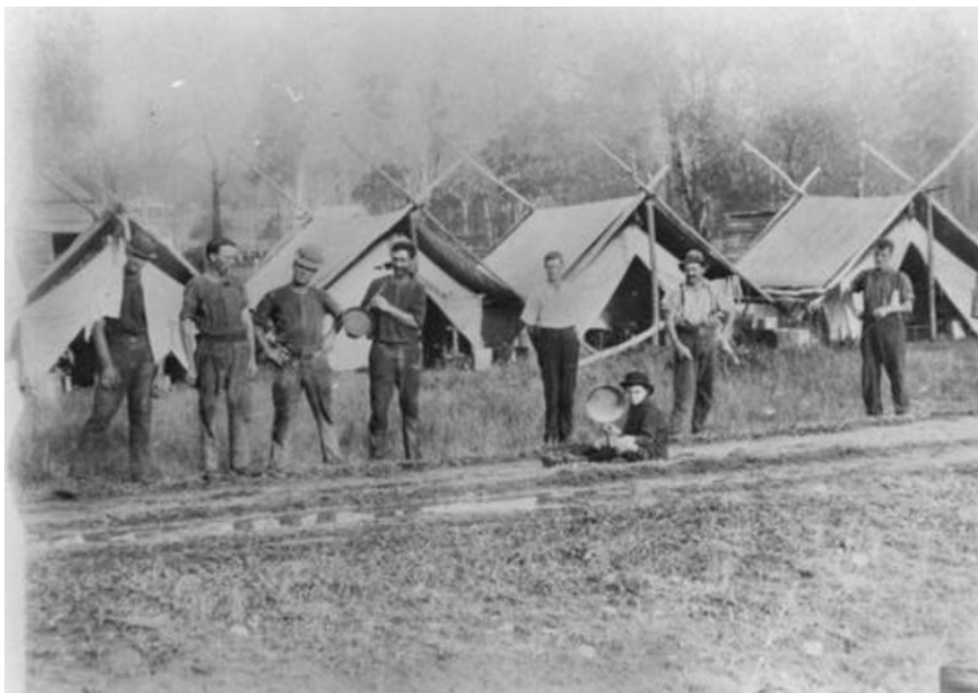
Figure 46: Railway fettlers' camp at Eudlo 1914 (John Oxley Library)
