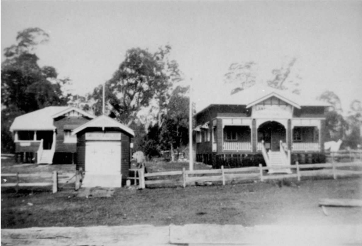
Figure 52: Landsborough Shire Council Chambers, c.1924 (Sunshine Coast Library).
