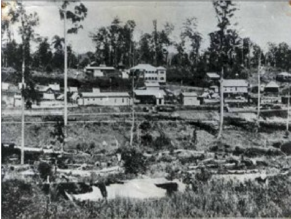
Figure 58: Palmwoods Station no date (Palmwoods.net.au)
