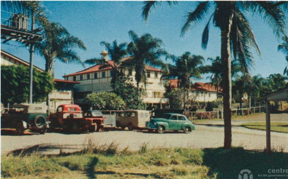
Figure 96: Section of the Nambour Hospital, c1958 (Centre for the Government of Queensland).
