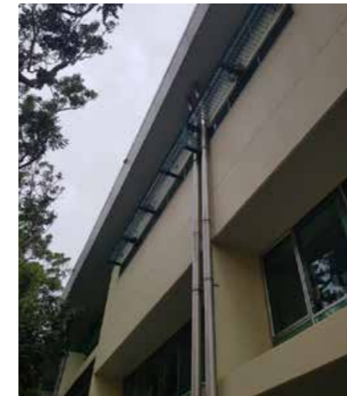
External Stormwater Downpipes
