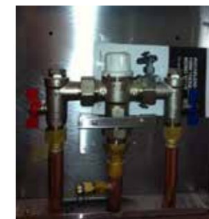
Typical Thermostatic Mixing Valve
