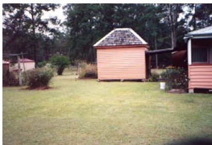
Dairy and Laundry, showing shingled roof.
