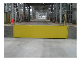
Figure 43 Lift and swing hinged flood gate - industrial (<u>www.psdoors.com</u>)
