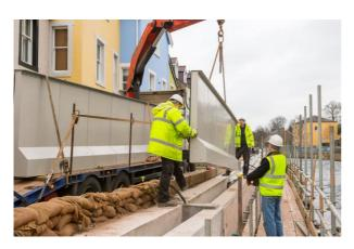
Figure 29 Large scale passive flood barrier system – panel installation A (www.globalfloodds.com)
