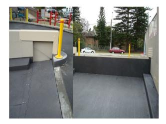
Figure 28 Flip-Up activated flood barrier for basement carpark entrance example (www.floodingsolutions.com.au)
