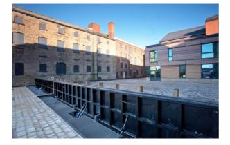
Figure 26 Flip-Up activated flood barrier example (<u>www.aquobex.com/products/flip-upbarrier</u>)
