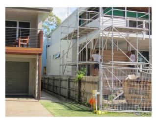
Figure 16 Highset house construction with raised lower floor level
