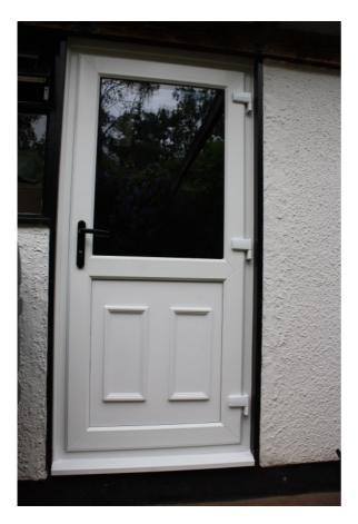
Figure 41 Domestic flood door application (<u>www.doorfactory.co.uk</u>)
