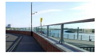
Figure 36 Permanent glass flood protection panels – public flood defence system application (www.floodcontrolinternational.com)
