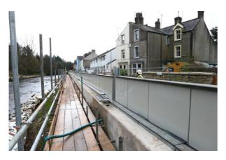
Figure 30 Large scale passive flood barrier system – panel installation B (<u>www.globalfloodds.com</u>)
