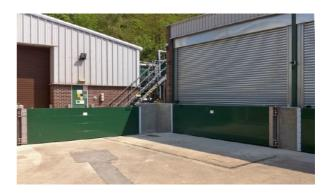
Figure 44 Lift and swing hinged flood gate (www.floodcontroltechnology.com.au)
