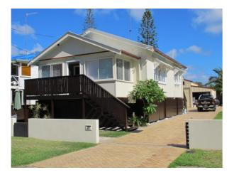
Figure 15 Raised timber house with understorey screening
