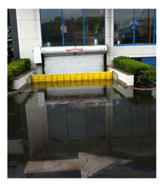
Figure 33 Passive flood barrier system – basement carpark entrance (<u>www.flood-barriers.com</u>)
