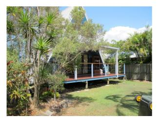
Figure 12 Light weight house construction raised above target flood level
