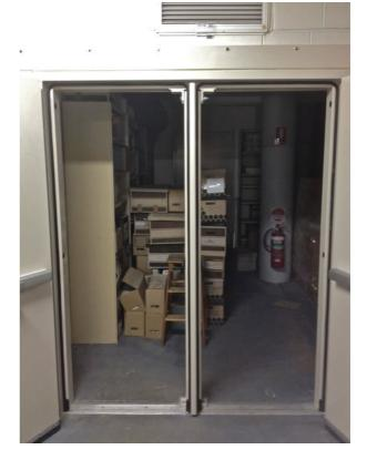
Figure 40 Commercial/Industrial flood door application (<u>www.floodingsolutions.com.au</u>)
