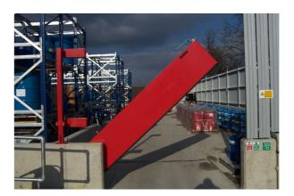
Figure 45 Side vertical pivoting flood gate (<u>www.floodcontroltechnology.com.au</u>)
