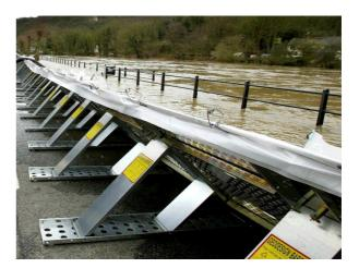
Figure 25 Temporary rigid flood barrier (<u>www.hydroresponse.com</u>)
