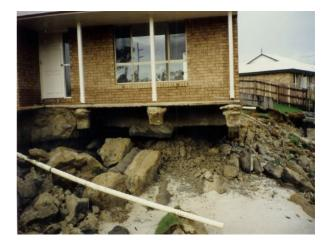
Figure 20 Eroded building footings from moving flood waters
