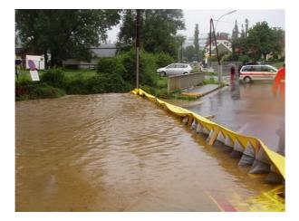
Figure 24 Temporary flexible flood barrier (<u>www.hydroresponse.com</u>)
