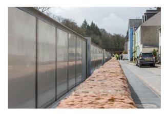
Figure 32 Large scale passive flood barrier system – panel engaged (<u>www.globalfloodds.com</u>)
