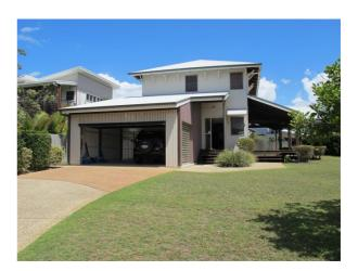
Figure 18 Suspended timber lower habitable floor level and second storey flood retreat area
