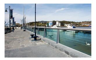
Figure 37 Glass flood protection panels (<u>www.careyglass.com</u>)
