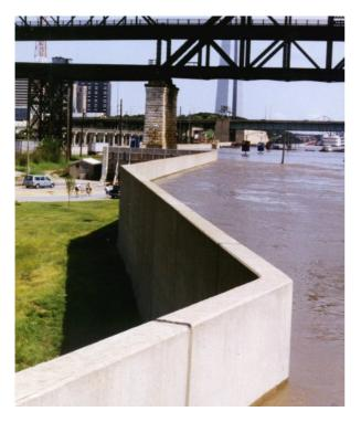
Figure 34 Permanent flood wall providing community protection (<u>www.coolgeography.co.uk/</u>)
