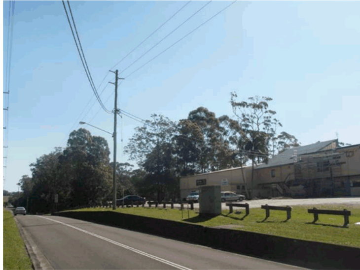
Figure 7 Services over and adjacent to Wises Road near clubhouse
