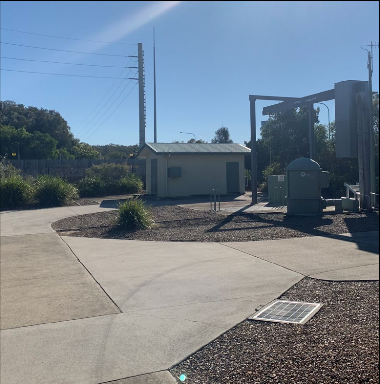
Figure 2 – Unitywater Infrastructure on Site
