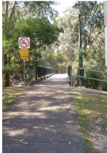
Foot bridge Esplanade Park across Mountain Creek
