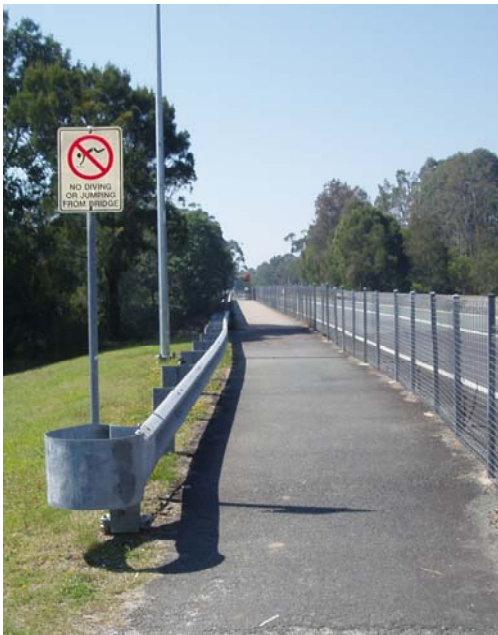
Footpath Prelude Drive Bridge
