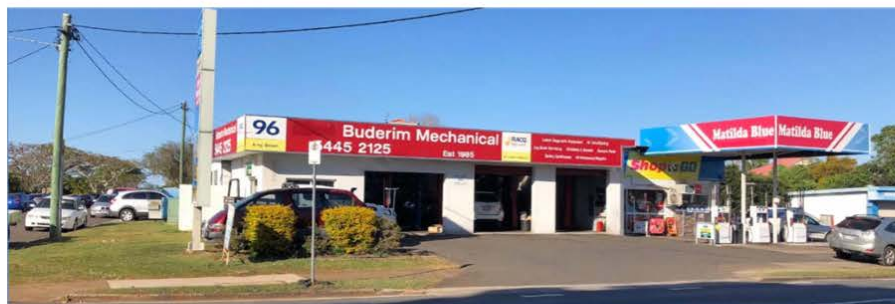
Photo 1 existing service station (King Street frontage)
