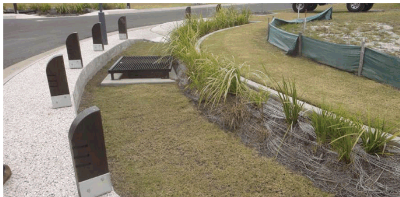
Photo 1 – Traditional concrete refuge plus kerb turn-out and forebay (Britinya) – not a desired outcome
