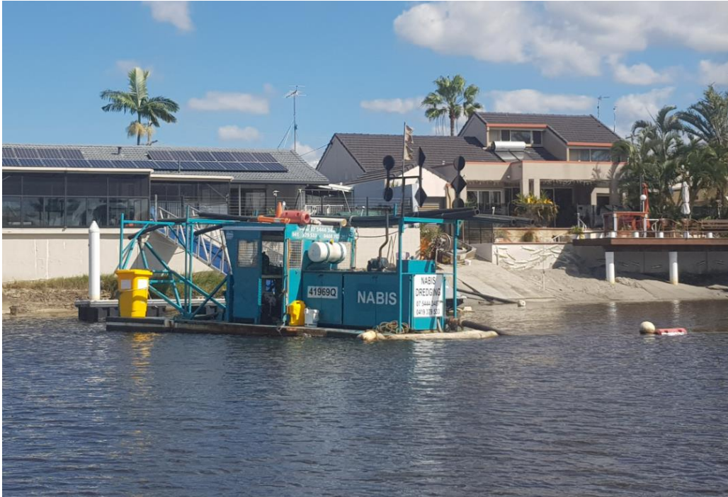
Figure 3-3 Dredging in progress to raise canal beach levels
