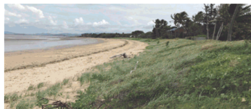
Buried geo-bag seawall at Zilzie, QLD
