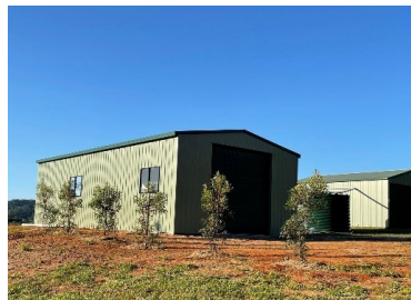
Figure 21: Image of existing Maintenance Sheds
