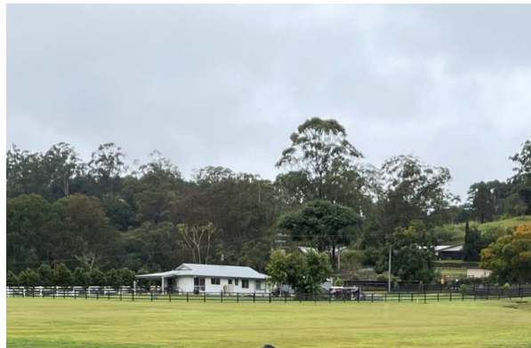
Figure 22: Image of existing Secondary Dwelling (to become Caretakers Residence)
