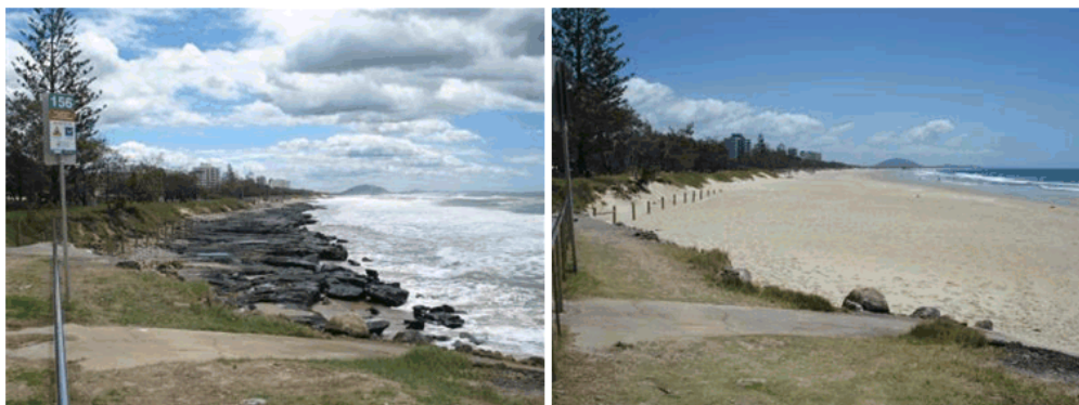
Figure 2-7 Before (left) and After (right) Maroochyde Beach Renourishment Project Stage One (photos courtesy of Birdon Pty Ltd)
