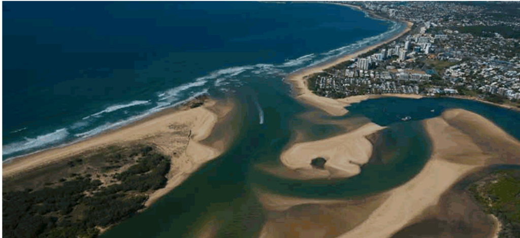
Figure 3-7 Maroochy River Mouth Dredging Works (photo courtesy of SCC, 2015)
