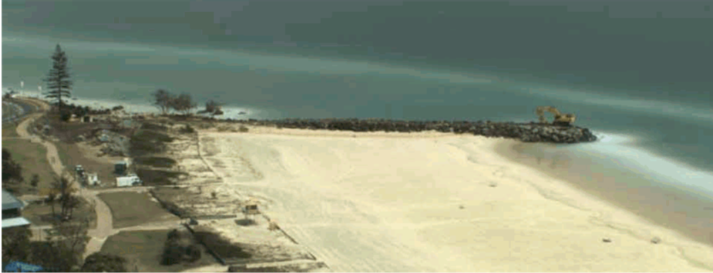
Figure 3-6 Kirra Groyne Extension Works (WRL Coastal Imaging, 2013)
