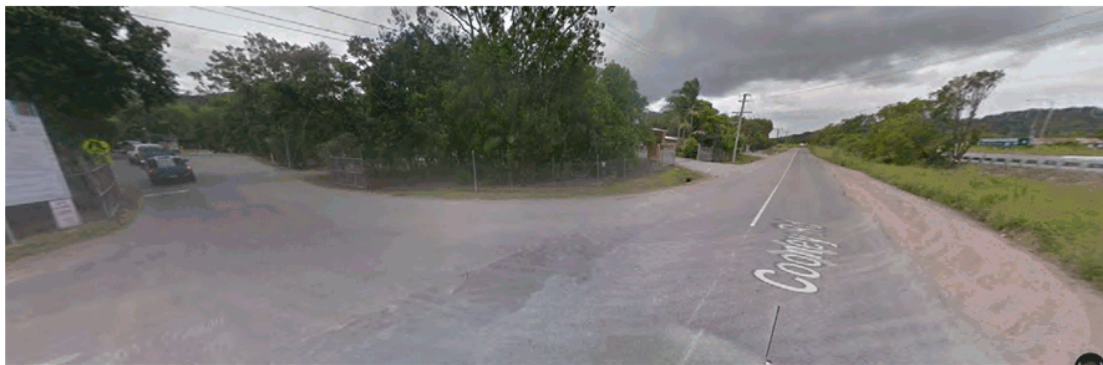
Figure 2.4: Existing landfill intersection (looking east)
