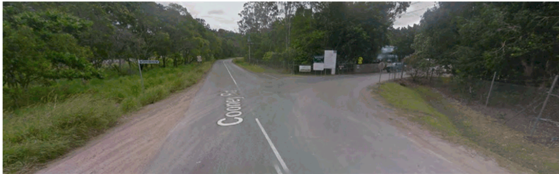
Figure 2.3: Existing landfill intersection (looking west)
