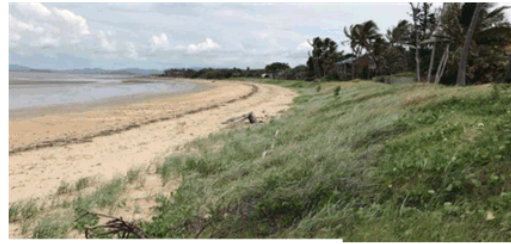
Buried geo-bag seawall at Zilzie, QLD
