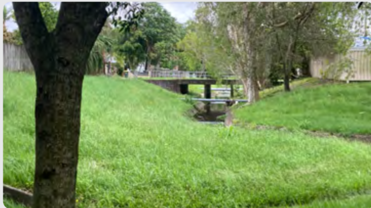
3 Creek contained in drain
