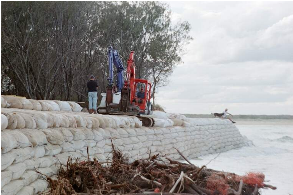
Figure 58: Geotextile seawall at the Maroochy River entrance
