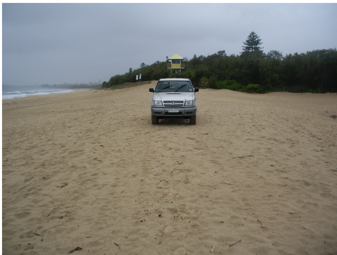
Figure 59: Berm constructed in August 2006 as part of entrance channel relocation
