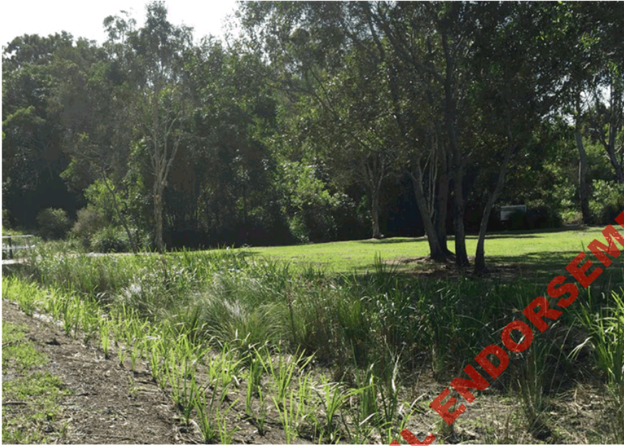
Figure 13 Better Open Channel –Free draining, densely planted, coil mat stabilisation during establishment, shading (source: Switchback Consulting)
