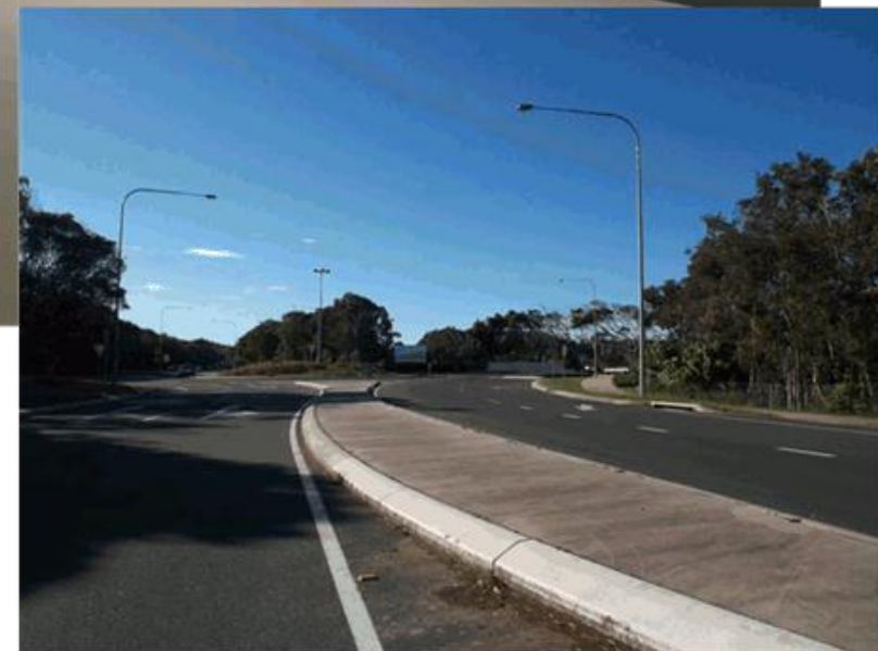
VP08b - David Low Way, existing roundabout
