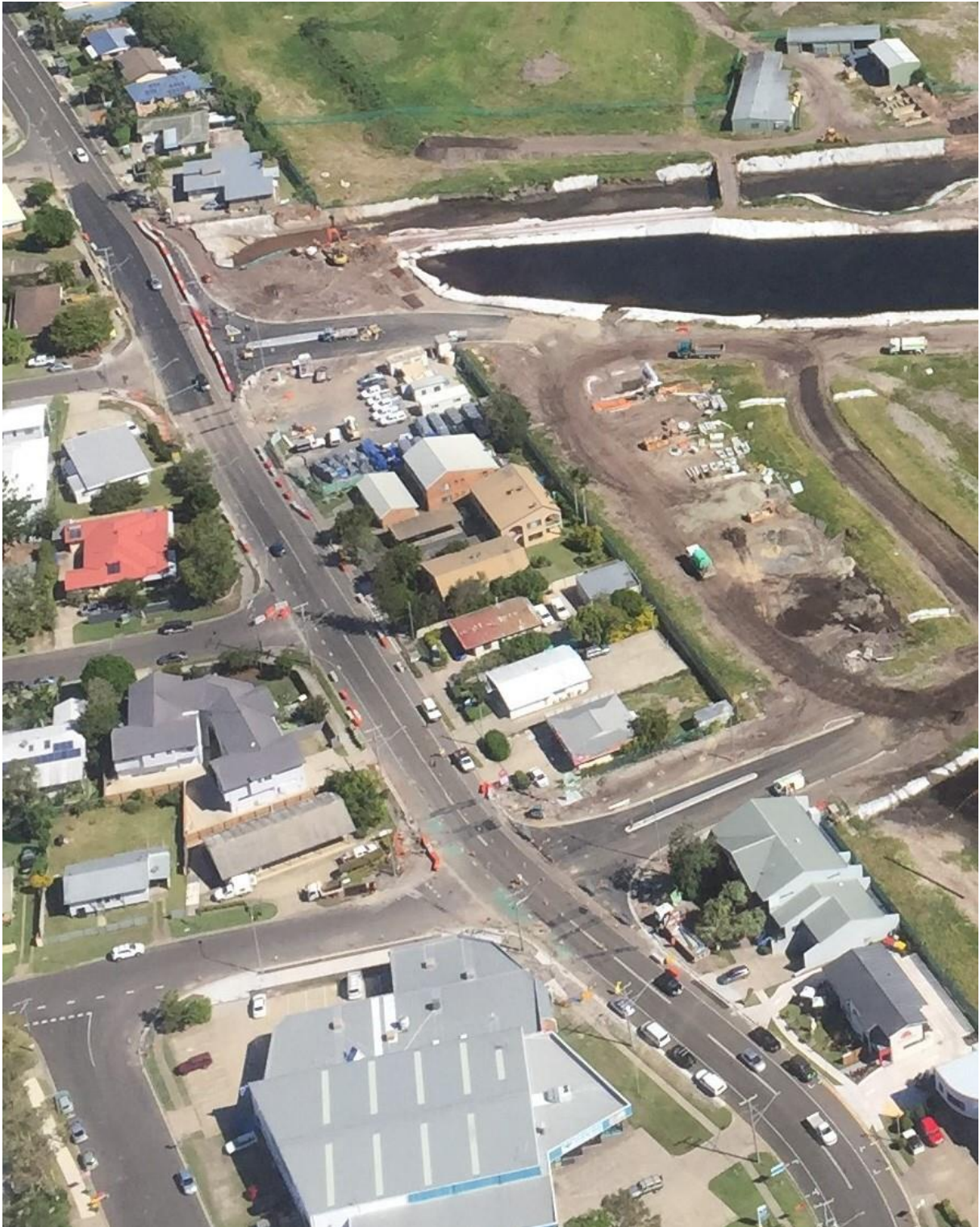
Fig 1. Maud Street Intersection works
