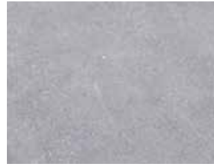
Coloured Concrete with Broom Finish.
