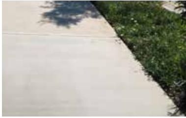
Footpaths: Plain grey concrete, broom finish
