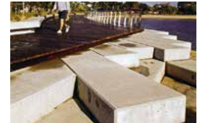
Access to Water: Formed concrete
