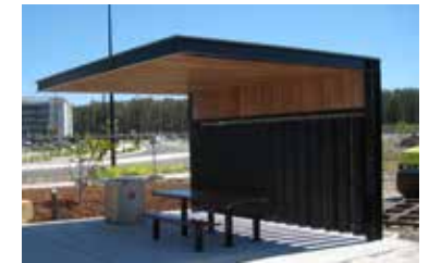
Shelters: Powder-coated steel framing and hardwood timber
