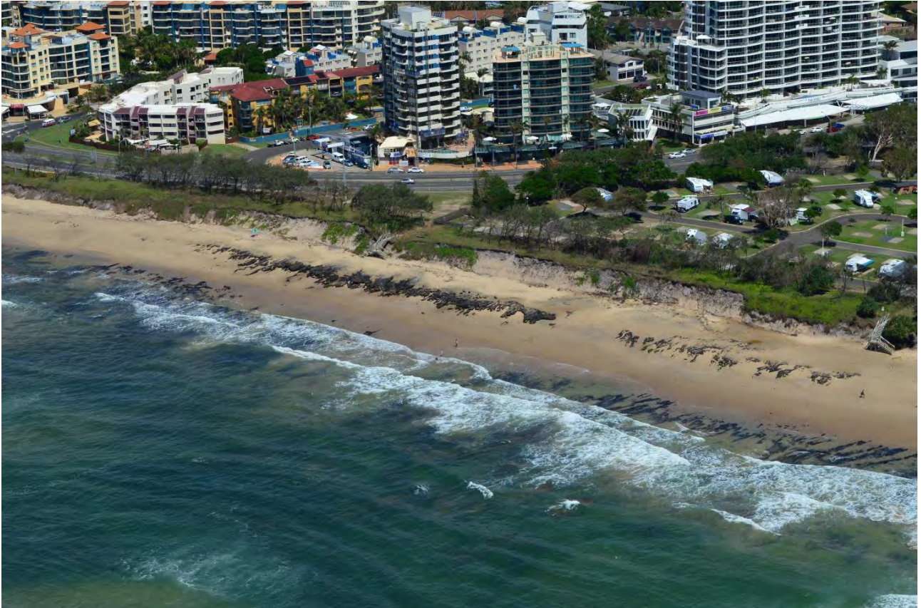
Figure 6.10: Maroochydore Beach erosion adjacent to the Seabreeze Holiday Park and Aerodrome Road/Alexandra Parade, March 2013
