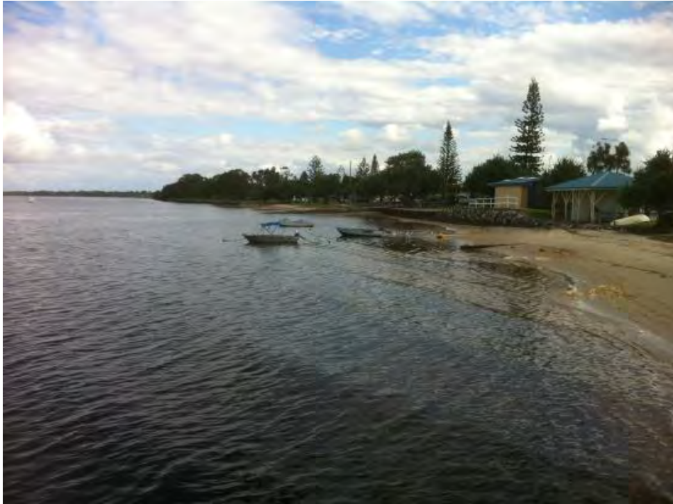
Figure 6.31: high recreation use beach south of Lamerough Canal showing narrow beaches and low sea walls (EMC1)
