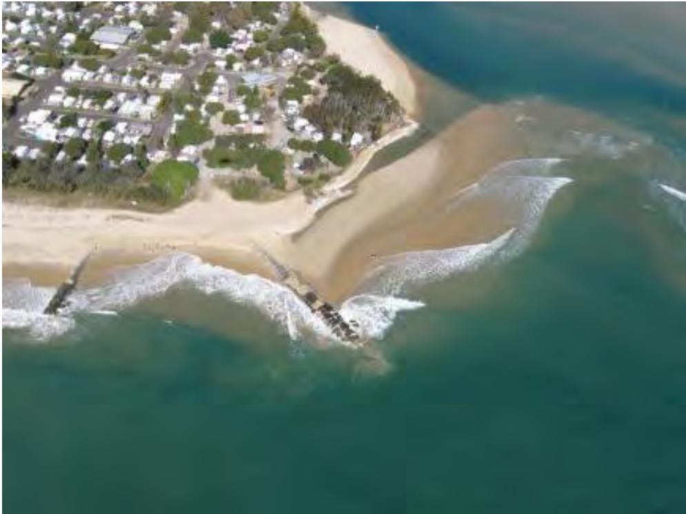
Figure 6.6: Maroochy River Entrance showing geotextile groynes.
