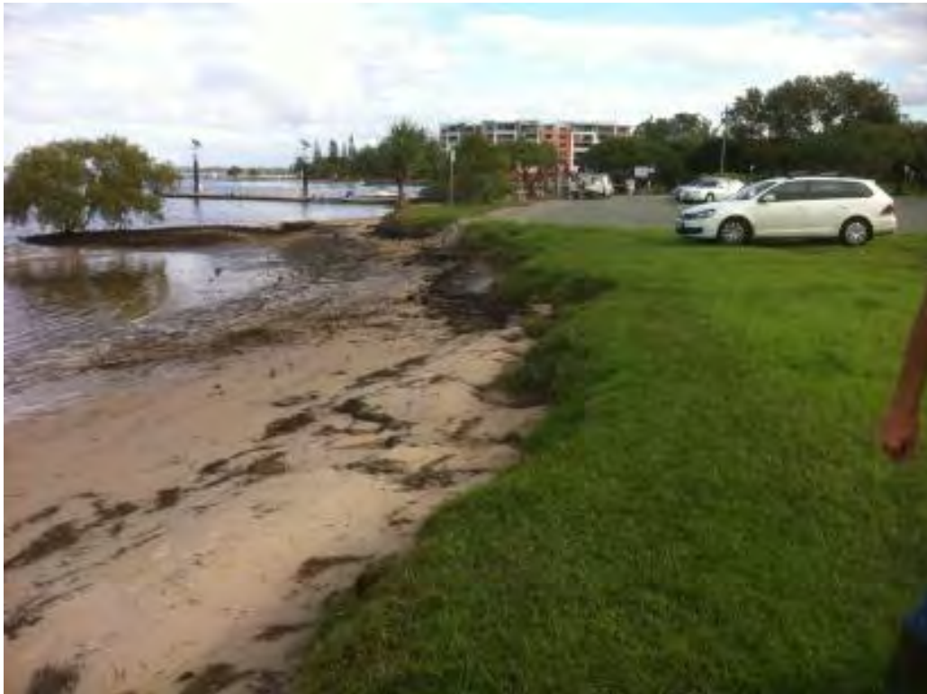
Figure 6.29: Photograph showing erosion of the shoreline at the Boat Ramp car park (EMC 3)
