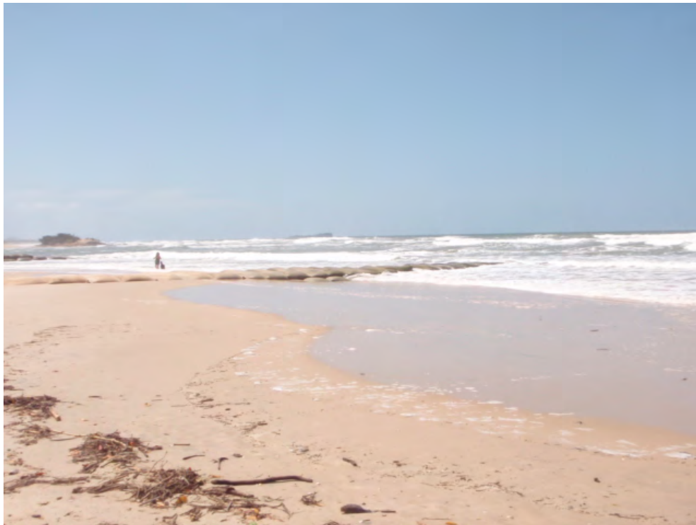
Figure 6.7: Geotextile Groyne at Maroochy River Entrance with Pincushion Island in the Background
