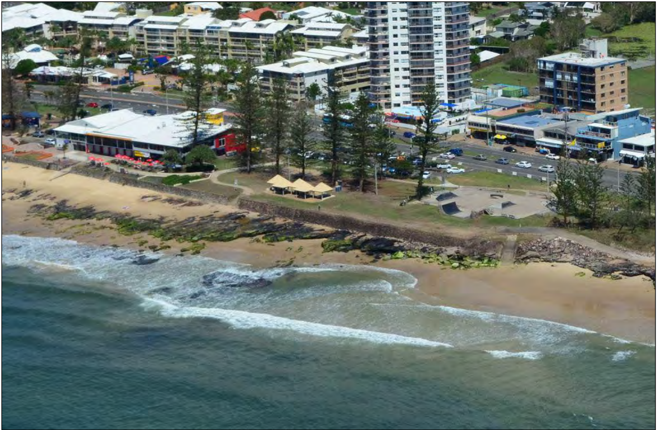
Figure 6.12: Exposed coffee rock at the toe of the Alexandra Headland sea wall
