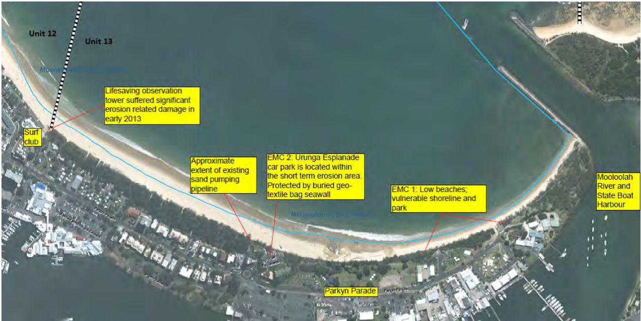
Figure 6.15: Annotated air photo locating the erosion management considerations for Mooloolaba Beach South
