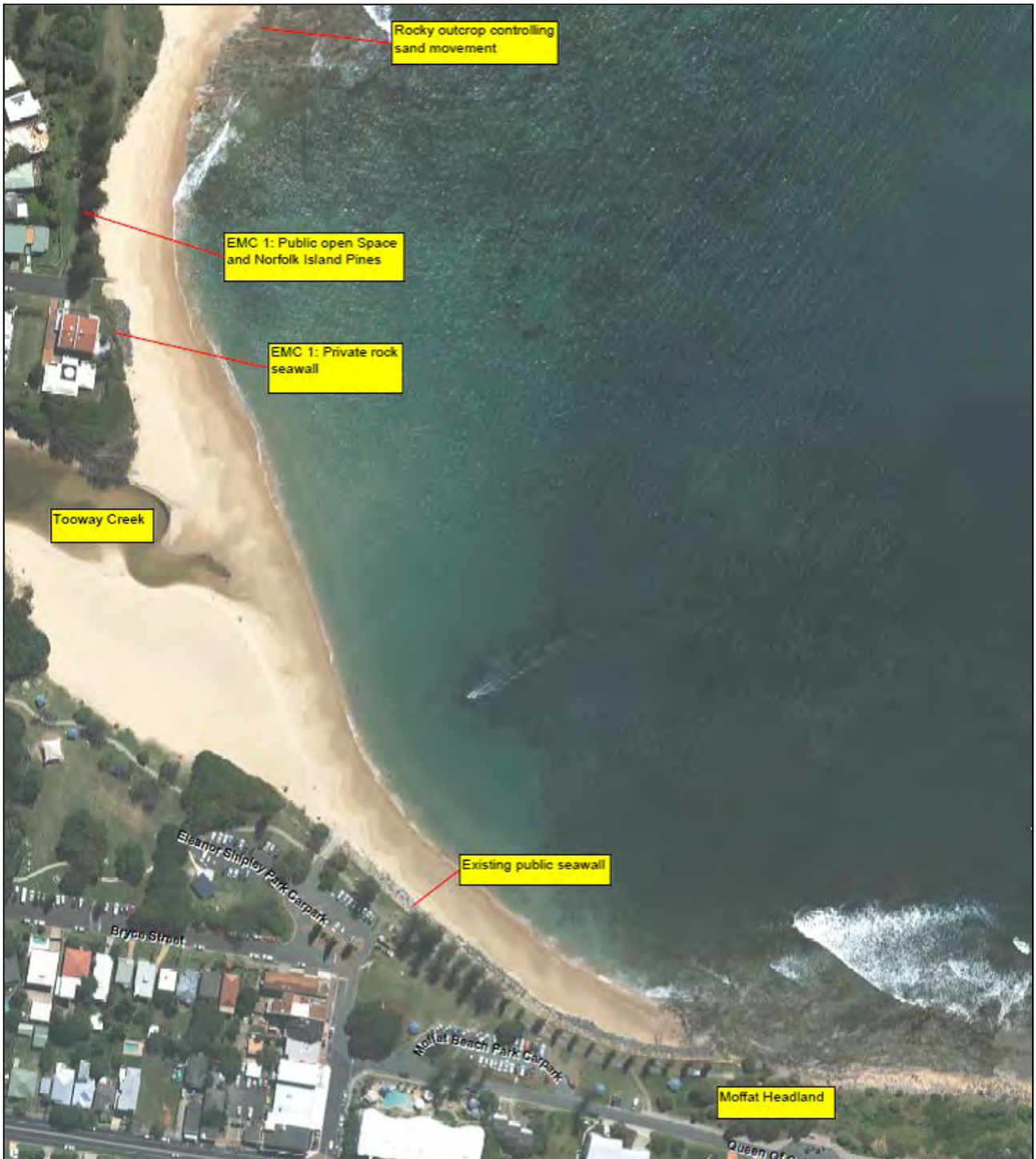
Figure 6.22: Annotated air photo of Moffat Beach showing the listed erosion management considerations
