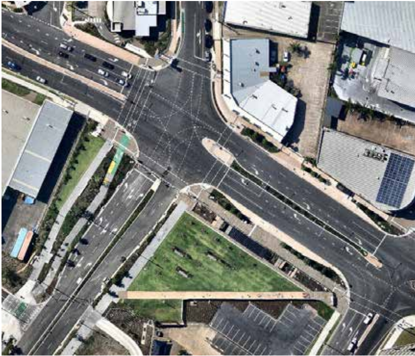
Completed Aerodrome Rd / Maud St intersection works by SCRC
