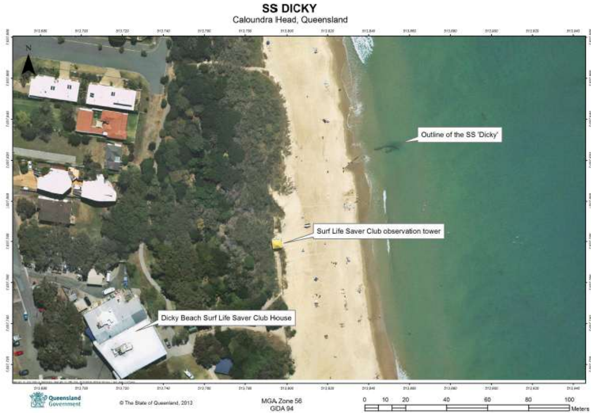
S.S. Dicky in relation to the beach and associated infrastructure (State of Queensland)
