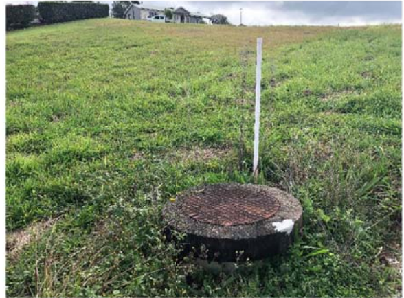
Sanitary sewer at subdivision to west of Site 1
