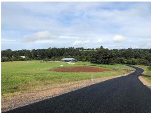
Porters Lane view of Site 2
