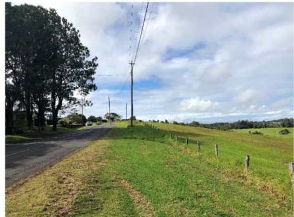
View of access road to Site 1
