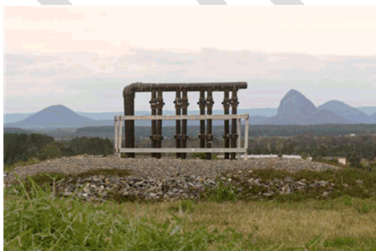
Image 15: Caloundra landfill gas manifold
