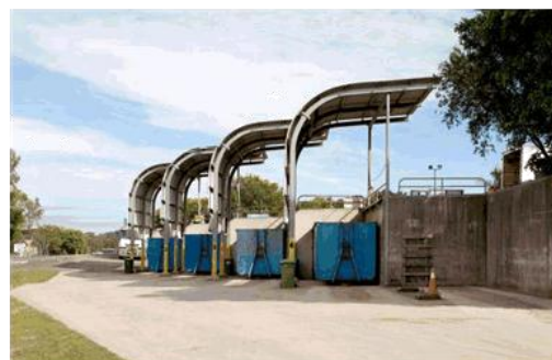
Image 14: Caloundra landfill transfer station
