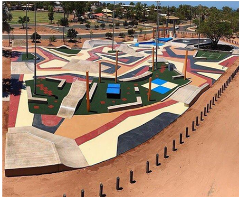
Figure 5 Onslow Skatepark, Pilbara WA
