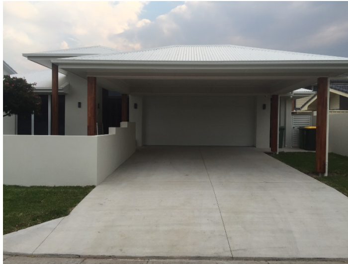
Front elevation of carport
