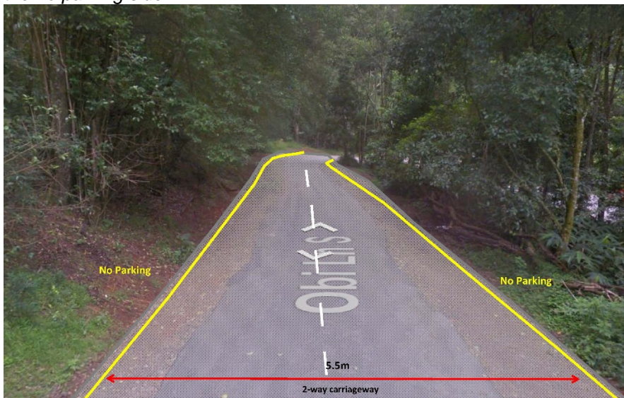
Figure 3. Option 2. Two way carriageway allows safe movement for vehicles. No parking. Bitumen surface would require widening.
