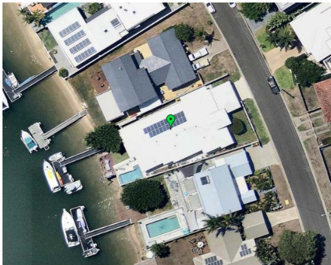
Aerial view of carport
