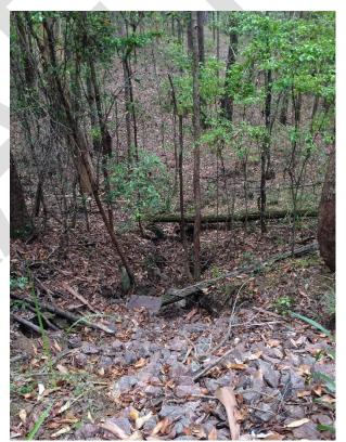
Erosion at rock chute along fire trail
