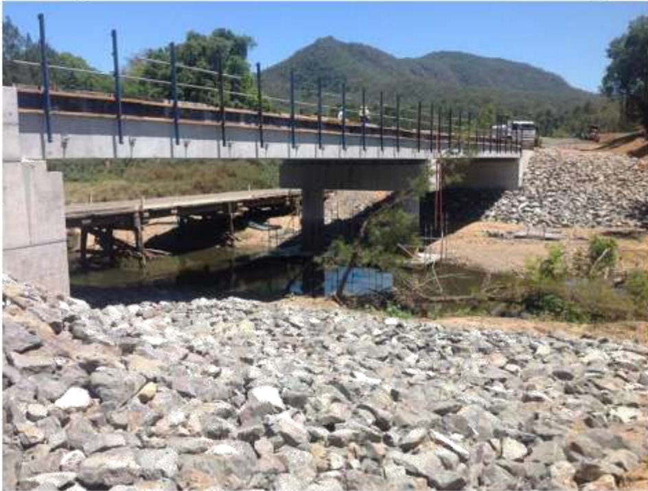
Above photo: View looking upstream.
