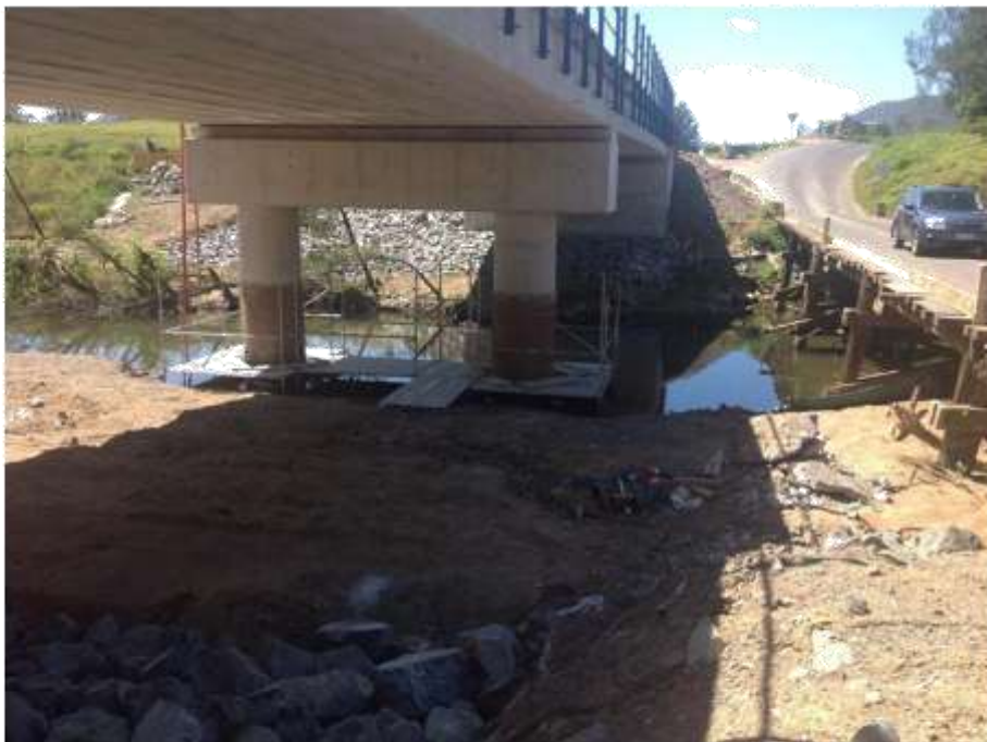
Above photo: View of both bridges looking south.
