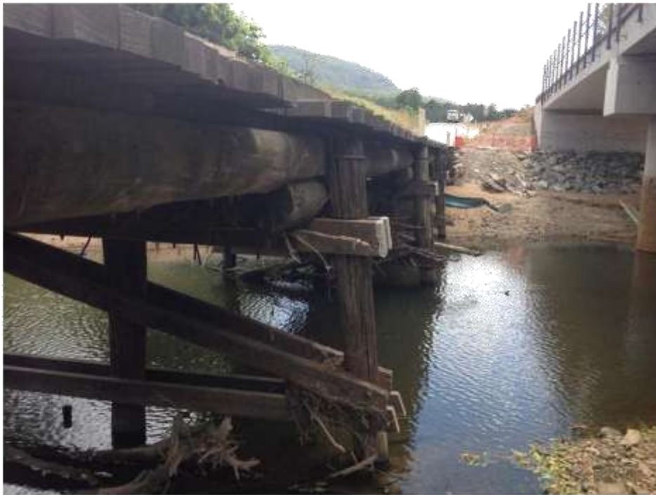
Above photo: View of existing Pickering Bridge looking north.
