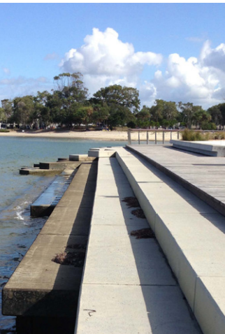
Waters edge: concrete revetment walls with some terracing to allow access to waters edge
