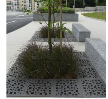
Tree grates: Powdercoated steel with patterned perforations
