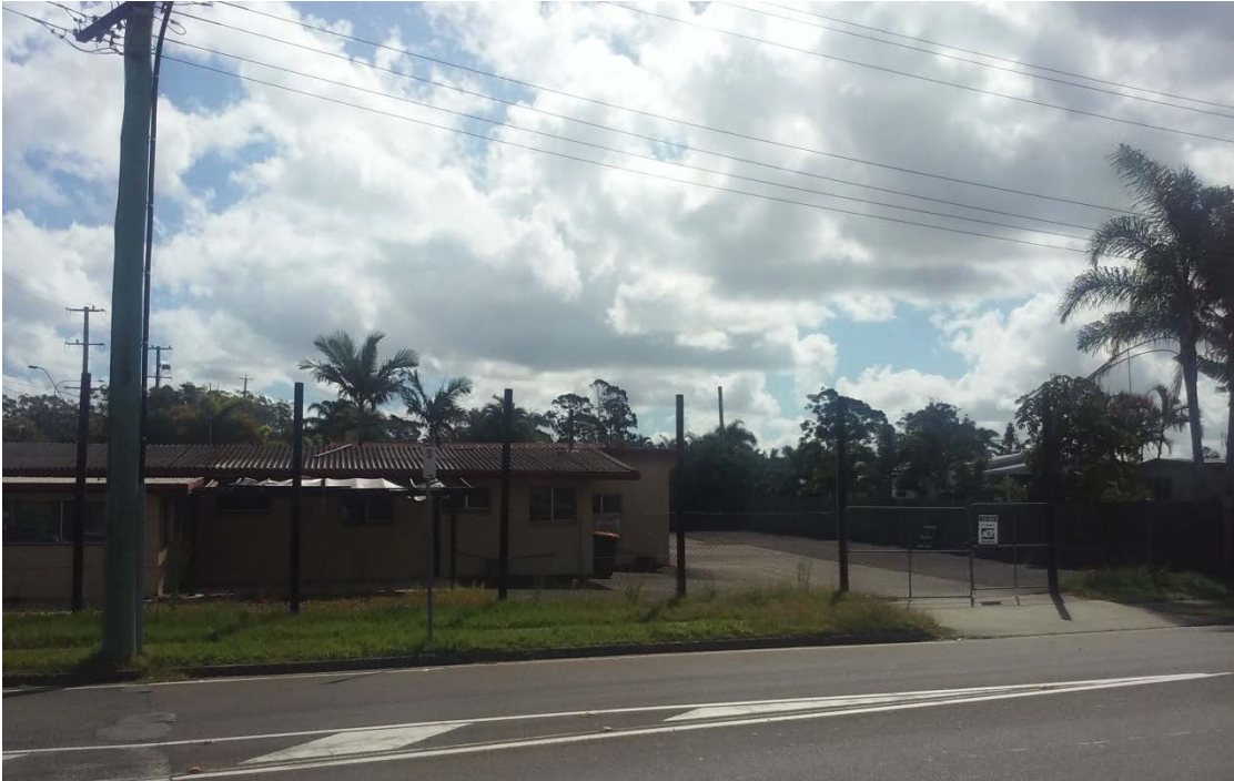
Existing (vacant) commercial use (06/04/2016)
