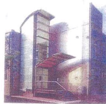
The creative use of materials helps to define the entry point and contribute to the architectural character of the building
