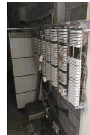
Figure 15 - Site Main Distribution Frame within Main Switchroom
