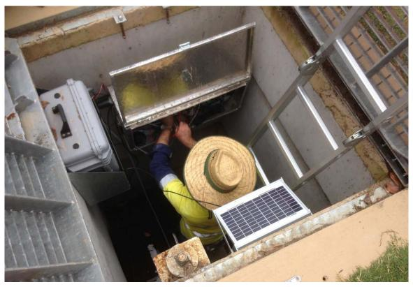
Figure 3 – Installation of Automated Water Sampling Equipment in Diversion Pit
