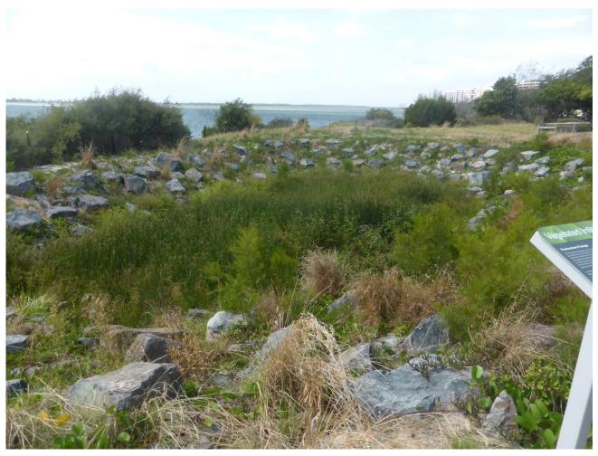
Figure 6 – Fully Established Vegetation in Earnshaw Street Infiltration Basin
