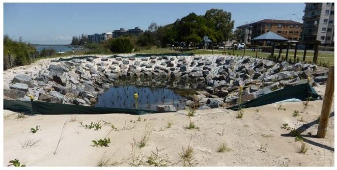
Figure 1 - Earnshaw Street Vegetated Infiltration Basin Installation (27-1-2015)
