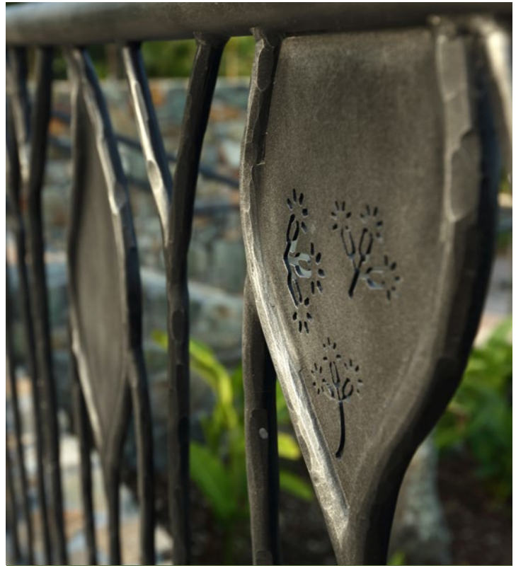
06 The material palette and construction techniques are inspired by the history, colours and textures of Palmwoods.
