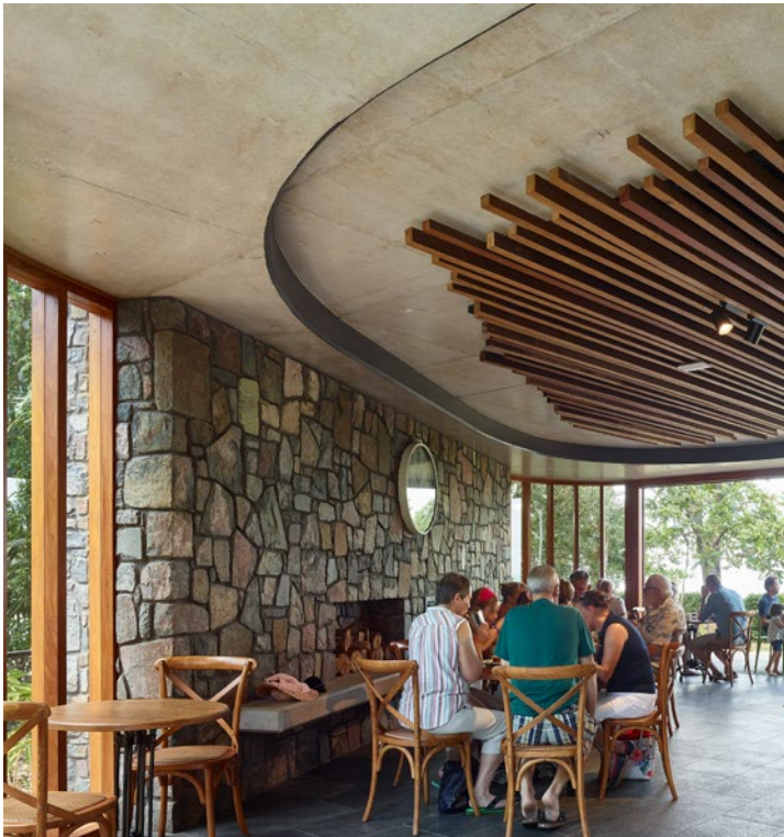
06 Locally sourced timber, Glasshouse Bluestone and Maleny bushrock, reflecting the character of the area, feature prominently in the building design and surrounding spaces. Gardens, incorporating 3000 plants grown from local seeds, establish a landscape setting for the building.
