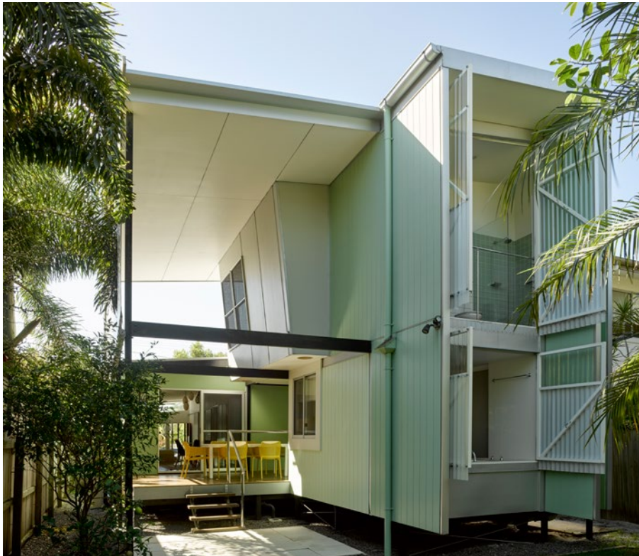
01 The inclusion of large windows and doors allow walls to open up and capture local breezes.
