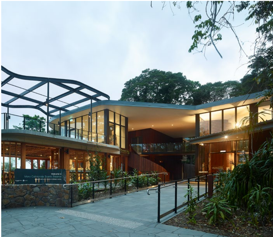
01 The building layout is in two parts linked by a breezeway that captures natural breezes. The building opens to the north to capture natural light and to the south to capture views.
