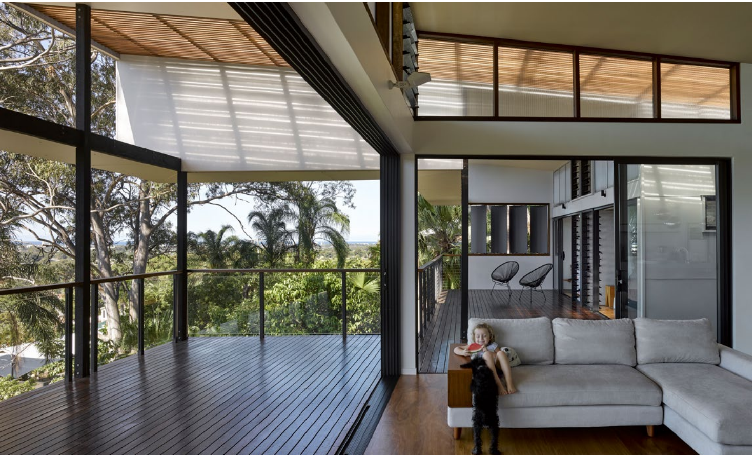
06 The ideas of 'Economical and robust' guided the choice of building materials which include galvanised steel, hardwood timber, polycarbonate, plywood, hardwood and fibre cement sheet cladding. The choice of material colours and textures reflect the natural colours and textures found on the site, in and around Buderim.
