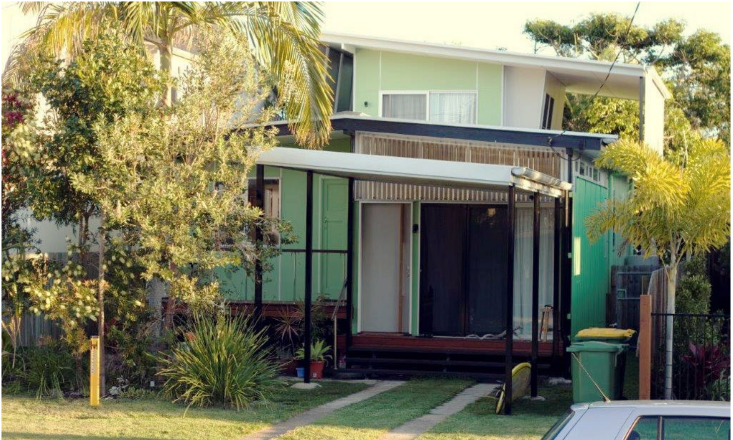
06 The simple low roof pitch of the extension is sympathetic to the scale and form of the existing house. The exterior colour scheme is a soft light green reflecting the era of the original fibro beach house and the natural landscape setting.
