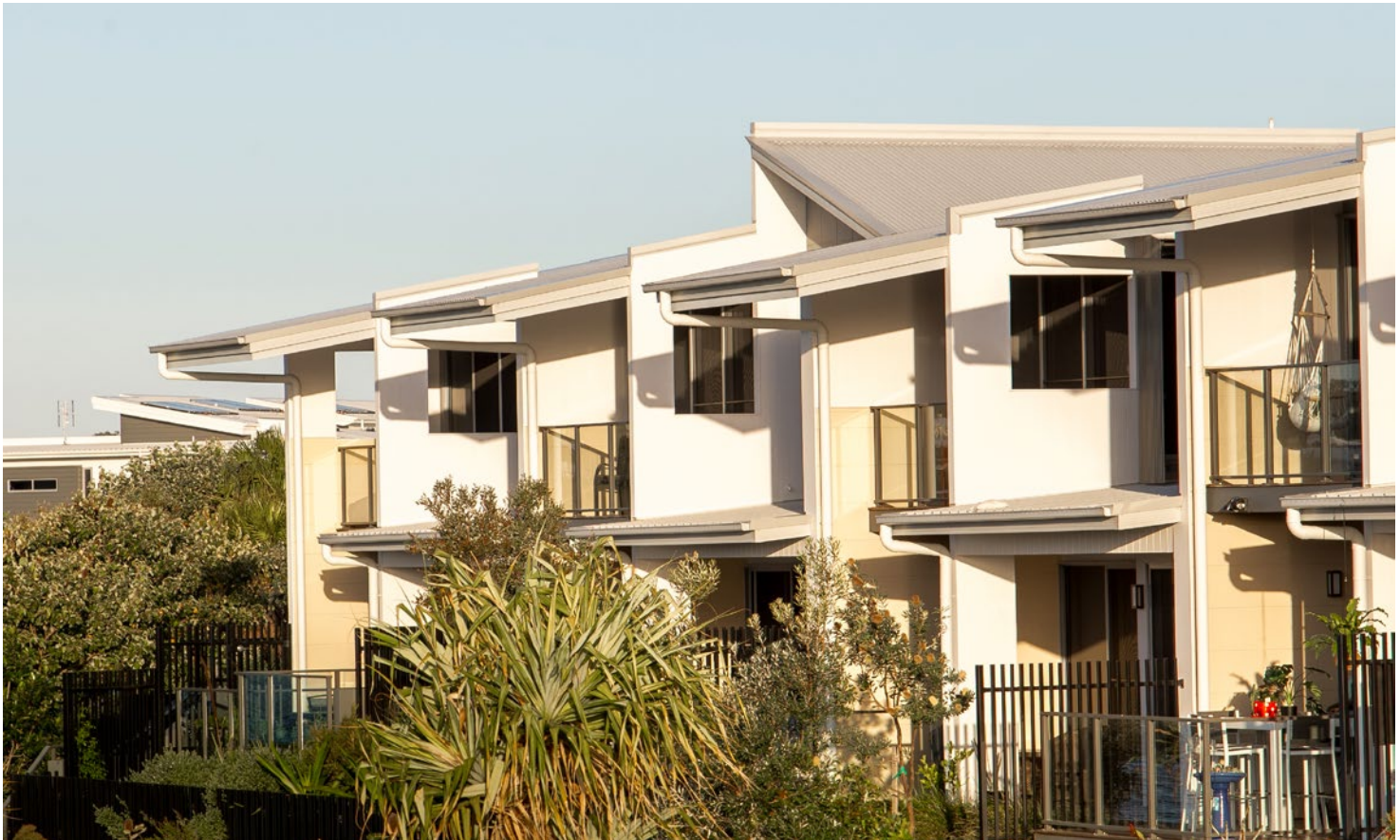
08 The development encourages community connection by locating individual gates to face public pathways and incorporating a private shared open central courtyard.
