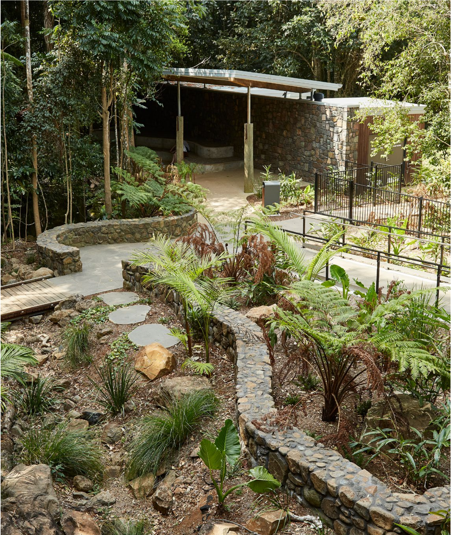
09 The building collects all rainwater and uses this to irrigate the Scenic Reserve. The stormwater design simulates natural systems to improve the site's natural hydrology. Sustainable water management includes collection and storage, bio-filtration and natural swales.
