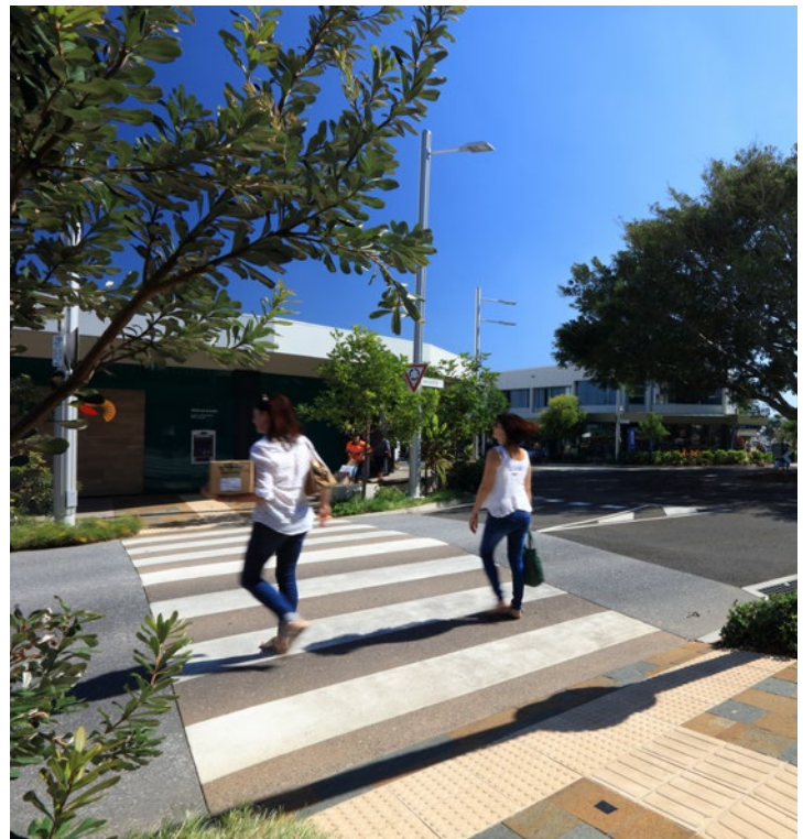
08 Flush kerbs provide a continuous accessible street surface for all pedestrians. Natural stone paving provides visual and textural way-finding at crossings and intersections.
