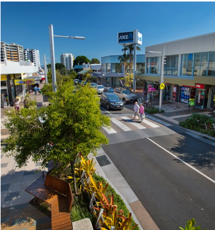
07 Telecommunication, gas, power and water services have been accommodated underground to 'free up' the street for pedestrians, shade trees, street furniture and cafe seating.
